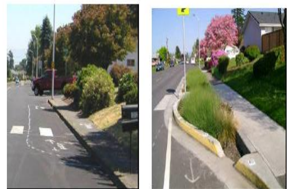
Before NIE Fremont Stormwater Curb Extension After.
