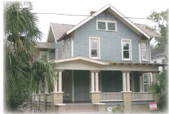
Green Restoration Project on 6th Street
