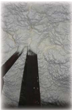
Spray foam insulation in attic
